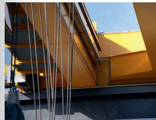
Kranbrücken in Parallelstellung Crane girders in parallel position
